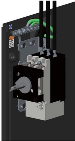
Fig. 4-13: Connection of the Primary Power Supply Cable
